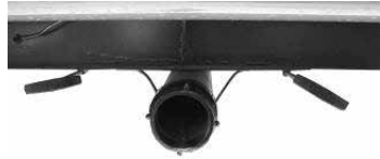
Black/Grey Tank Drain and Valves
